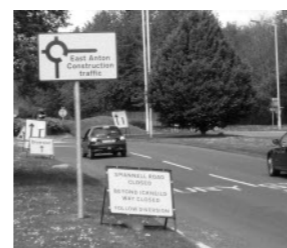
Road signs improved
