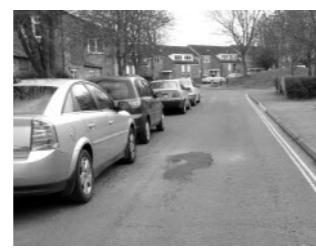
Potholes repaired
