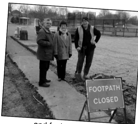
and footpath repaired as we visited the area
