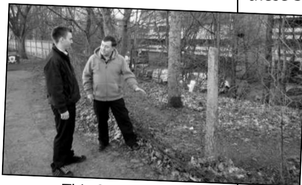
This fence is being repaired
